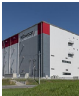
E17 REDWOOD Narita Distribution Centre
