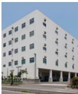
E8 Shin-Narashino Logistics Center
