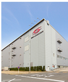
E9 Kawagoe Logistics Center
