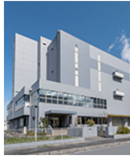
E15 Hirakata Nagao Logistics Center
