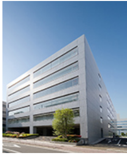
B8 UUR Toyoko Building
