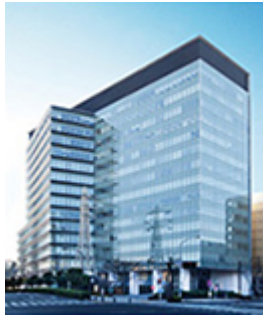
B37 ARENA TOWER
