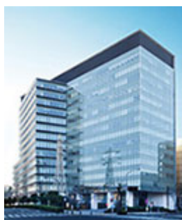
B37 ARENA TOWER
